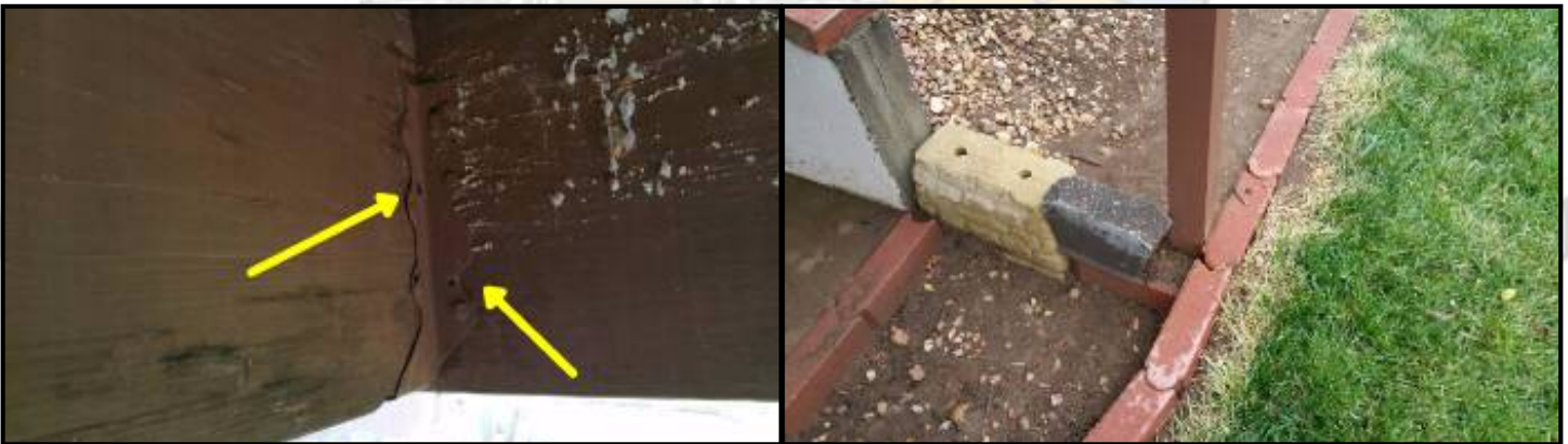
Missing nails in the joist hangers.
