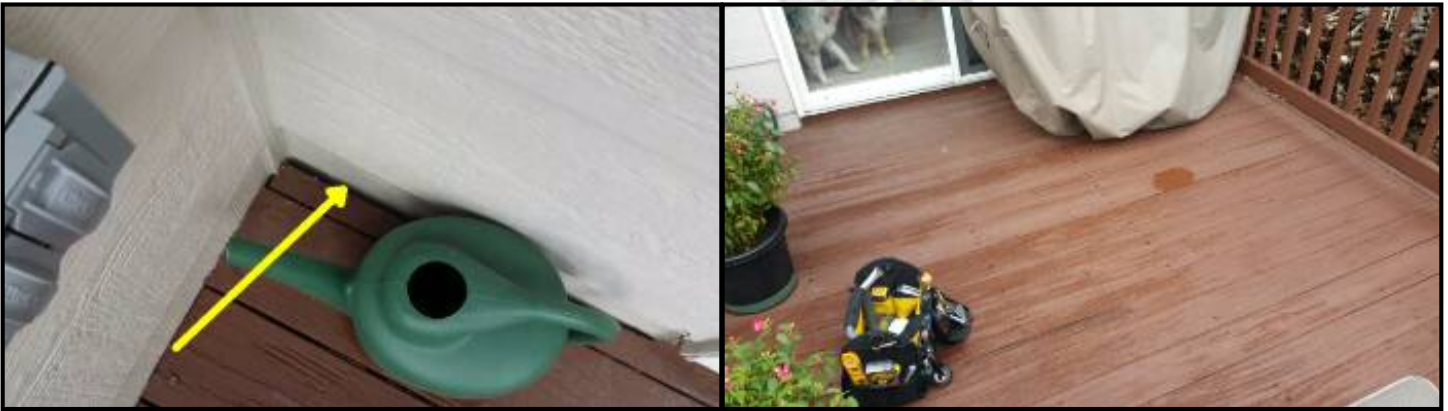
Missing flashing.
